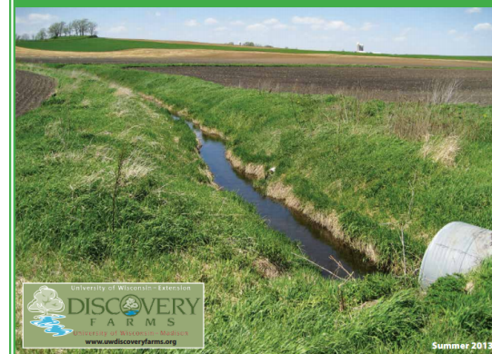
Figure 1: Tile outlet with a rodent guard.
