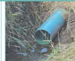
Figure 1: Tile outlet with a rodent guard.
